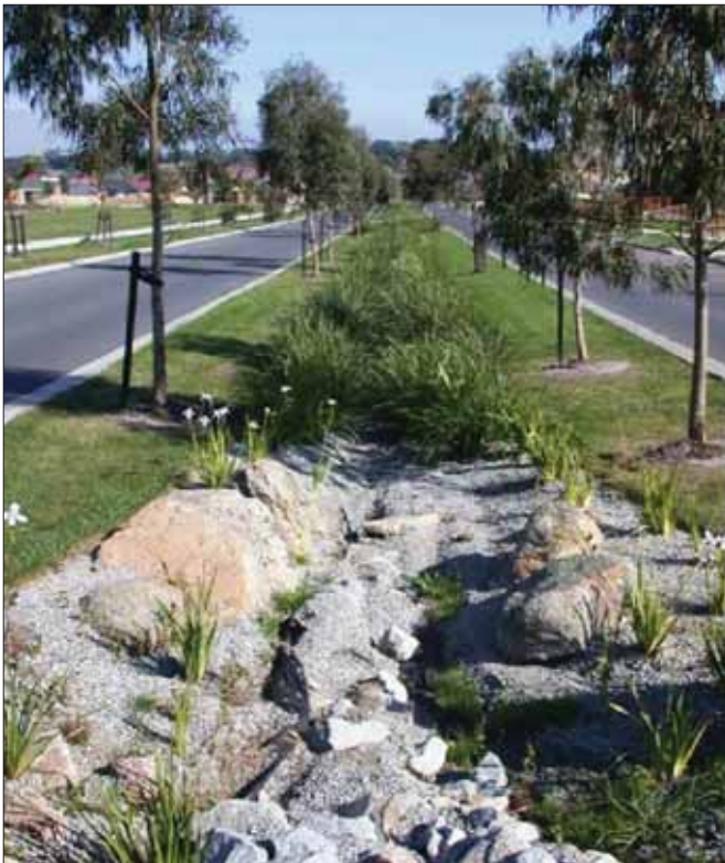
Figure 19. Bioretention system at Lynbrook Estate ( www.wsud.org )
