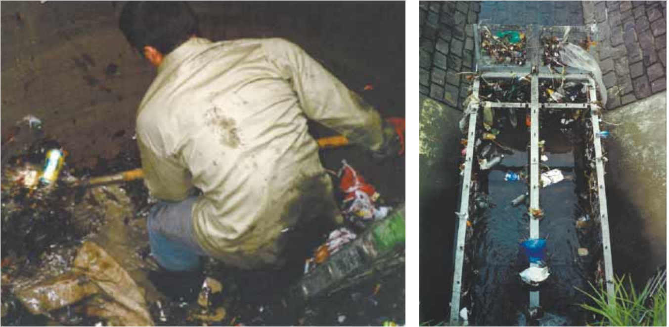
Figure 13. CRCCH Research into Urban Stormwater Gross Pollutant Composition and Trap Technology (courtesy Dr Robin Alison)
